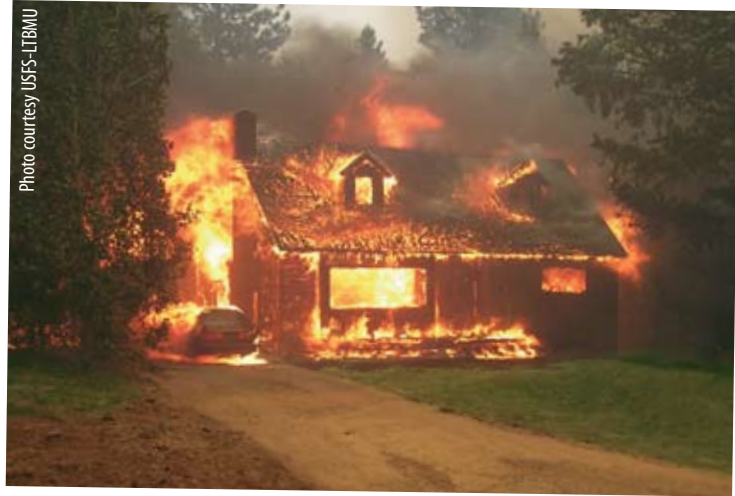
This house was ignited by burning embers landing on vulnerable spots. Notice the adjacent forest is not burning.
