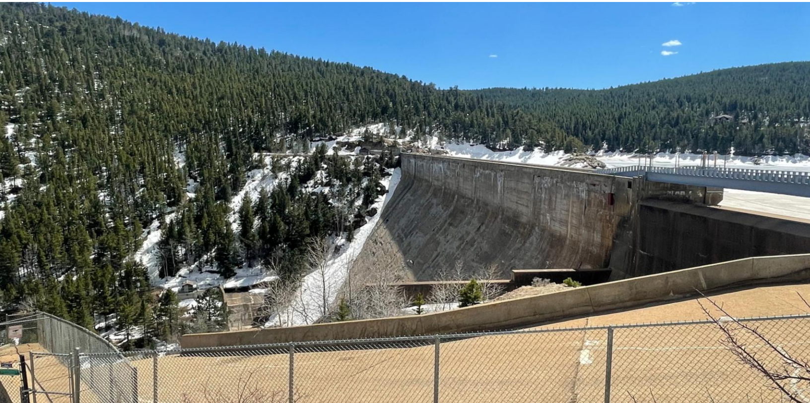
Figure 8: Barker Dam and Reservoir. Photo Credit: Boulder Watershed Collective
