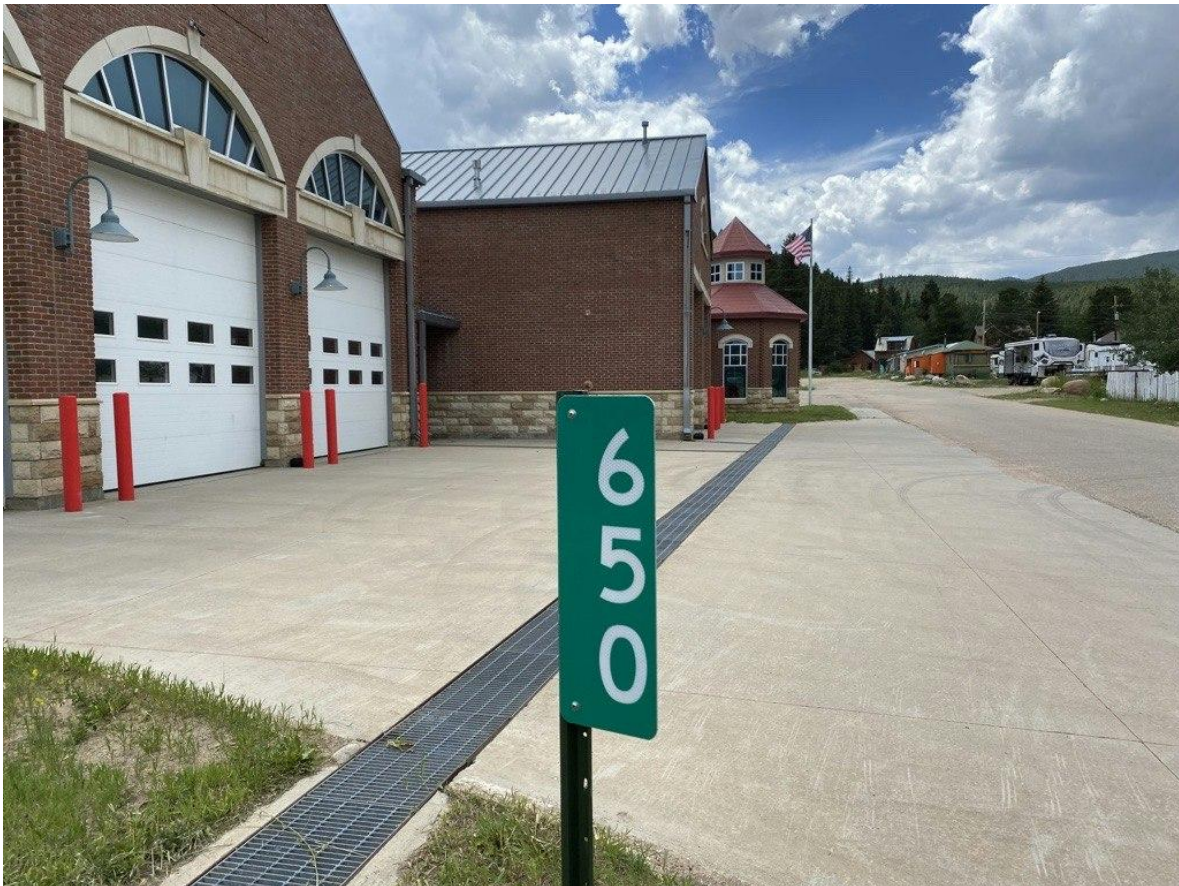
Figure 31: The new address sign out front of Station 1. Source: NFPD
