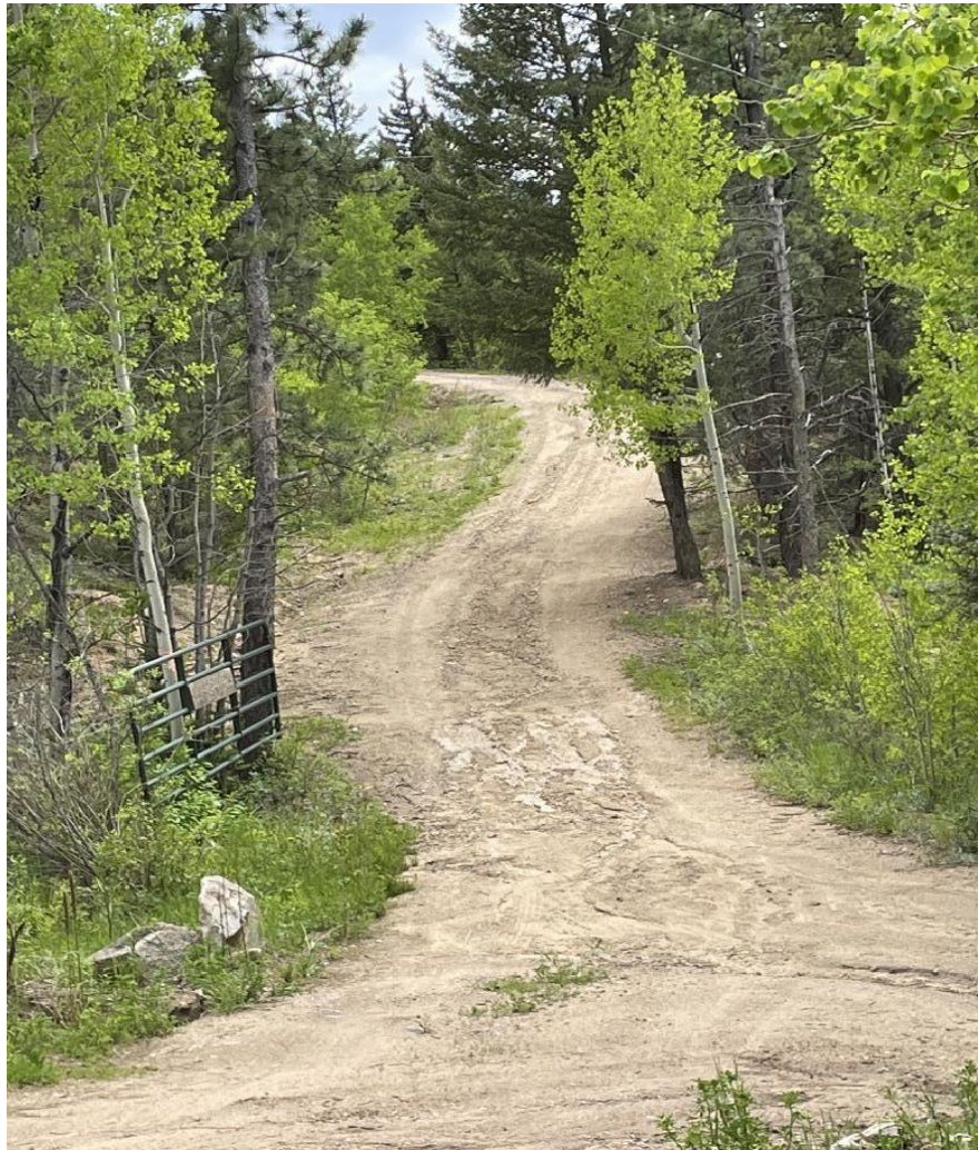
Figure 32: Many driveways within NFPD/TFPD do not meet current access requirements and pose safety issues that are difficult to mitigate. Long, narrow, and steep driveways lacking turnarounds, with dense trees overhanging the road, can create challenges for emergency response vehicles during wildfires.
